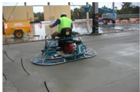
Figure 14.5 – Power Floating in a Regular Pattern
