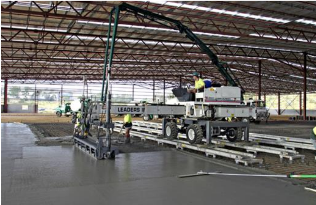
Figure 14.2 – Typical Machine-mounted Beam Screed
